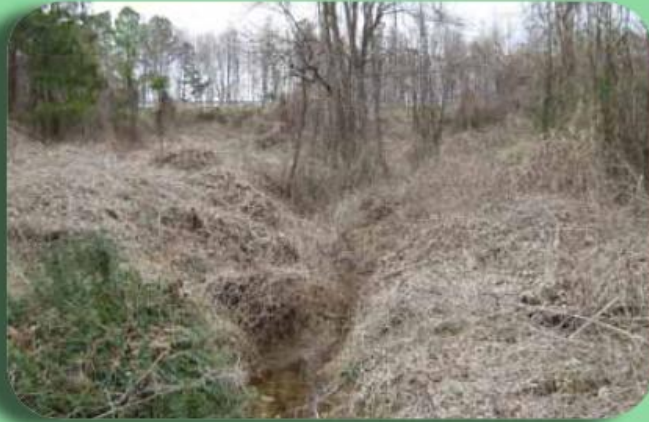
Torrence Trib #2 at I-77 before stream restoration
