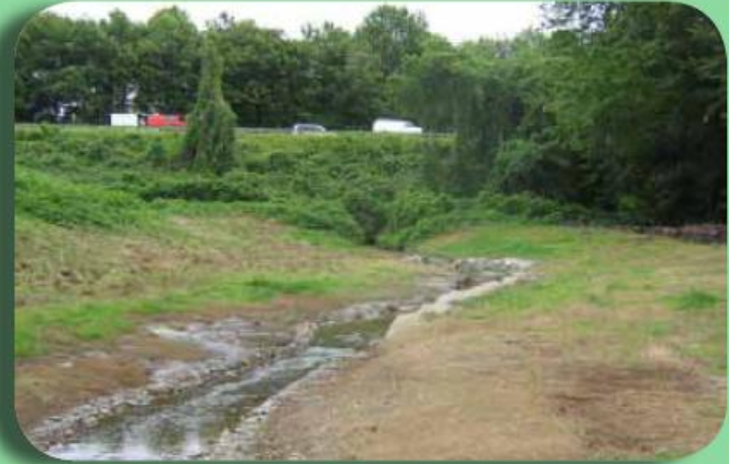
Same location, June 2010. The bed and banks have been restored. Next, native plants will be added to the banks and floodplain.
